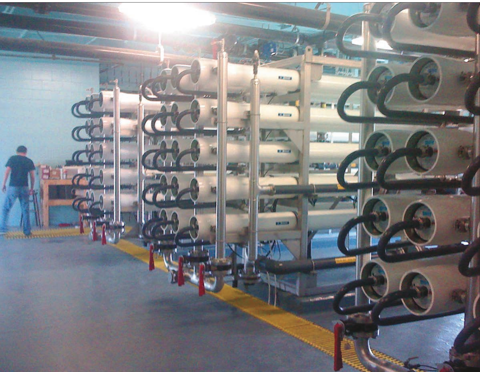
Example of Brackish Water RO Facility
